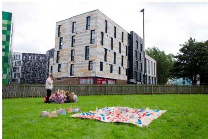
Photo 1: The Shield Development
